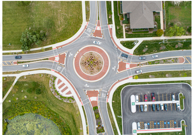
Ravinia Avenue Roundabout | Orland Park, IL
